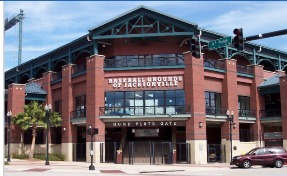
Electrical, Video and Sound installation performed by graduates of the program working for a member contractor.
